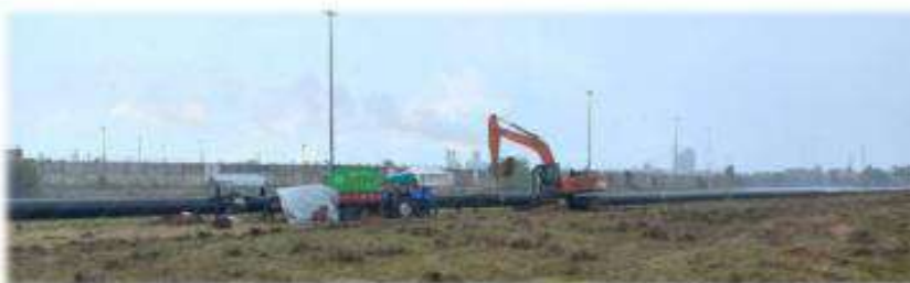
Setting up slurry pipeline
