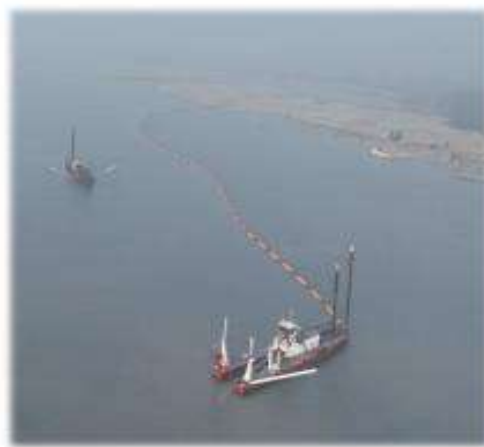
Dredging work underway at Jatadhar
