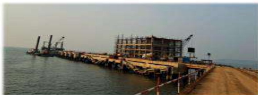
LPG construction at Jaigarh Port
